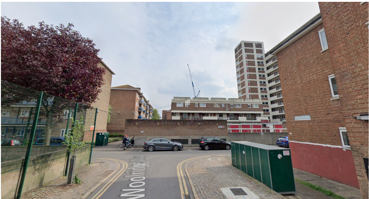
Garage Structures on Woolridge Way
