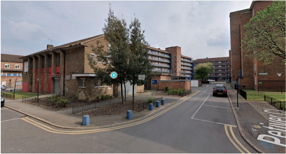
Looking south down Petiver Close
